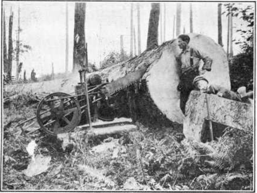
FIG. 1.—A small drag-saw outfit operated by one man. This is used to saw the big trees of the Pacific Northwest into firewood. It is mounted on skids and is pulled along for each new cut by means of a winch and cable.
